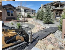
Special Access trees require an 8' opening for the larger equipment (not shown).
